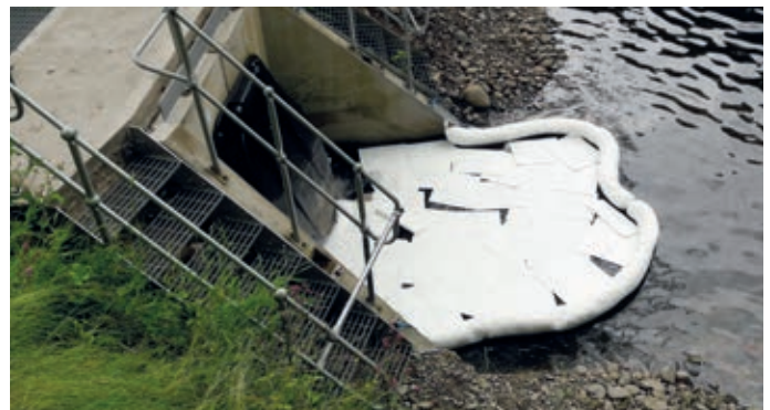
Measures deployed at a surface water outfall to mitigate the impact of a hydrocarbon pollution incident at an industrial estate
