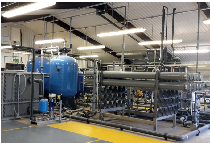
The testing facility at the Gorthleck Development Centre, showing the raw water storage tank, multimedia filters and ten membrane modules. Two testing bays can be seen in the foreground
